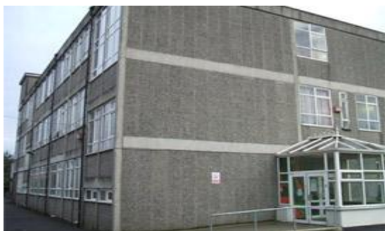
SCR - old School building at Ridge Road
