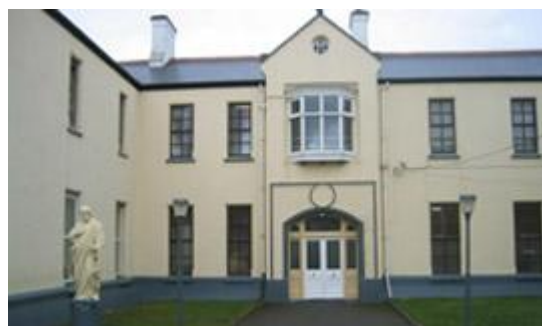
CBS - old School building at Tower Hill
